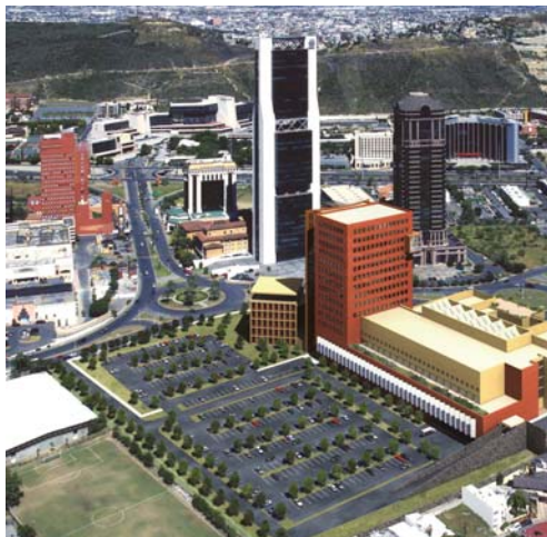
Site context. Image courtesy of Termo Técnica Quin.
