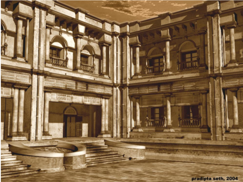
Old Courtyard Pradipta Seth
