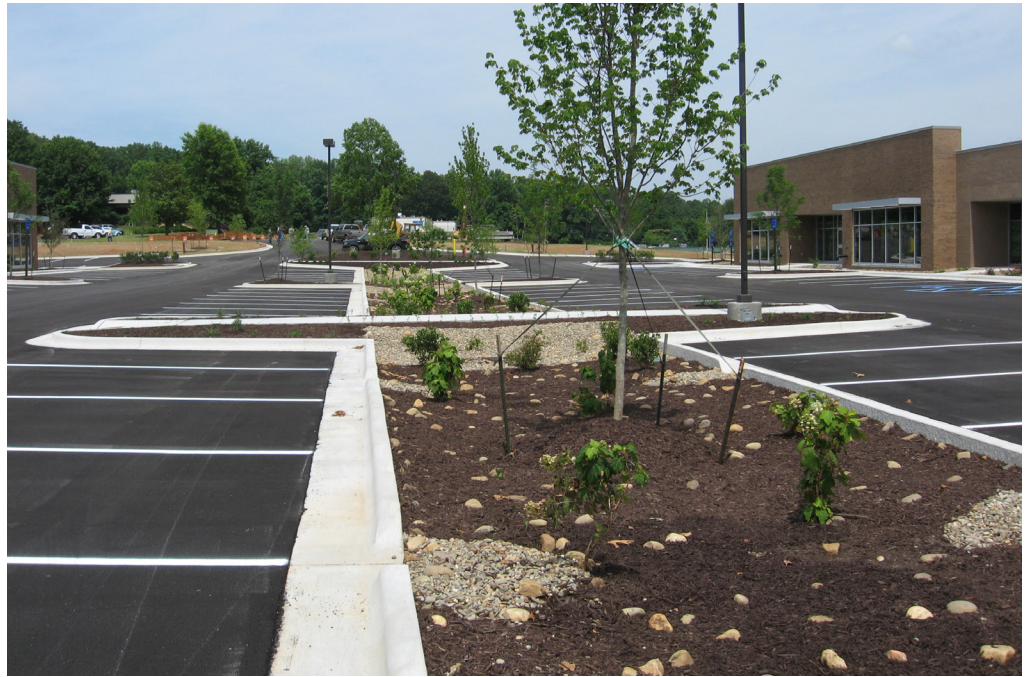
Civil 3D and Storm and Sanitary Analysis helped to plan and size individual gardens more efficiently saving time. Image courtesy of 4Site, Incorporated.
