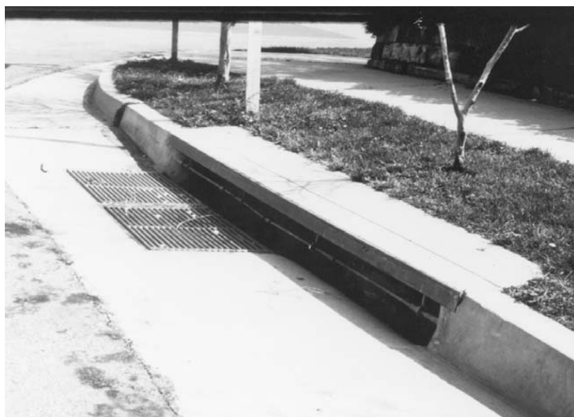
Figure 7.29 Combination sweeper curb opening & grate inlet
