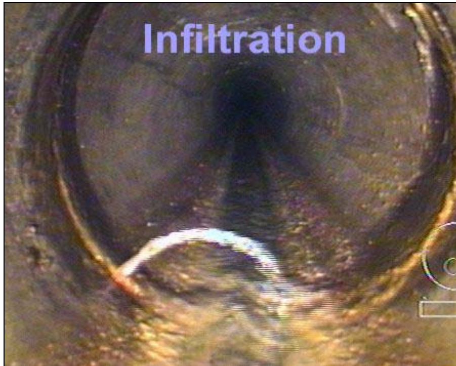
Figure 9.96 Example of infiltration into a sanitary sewer network (courtesy City of Surrey, Canada)
