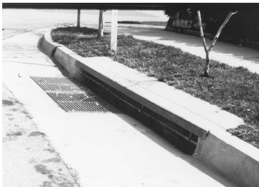
Figure 7.29 Combination sweeper curb opening & grate inlet
