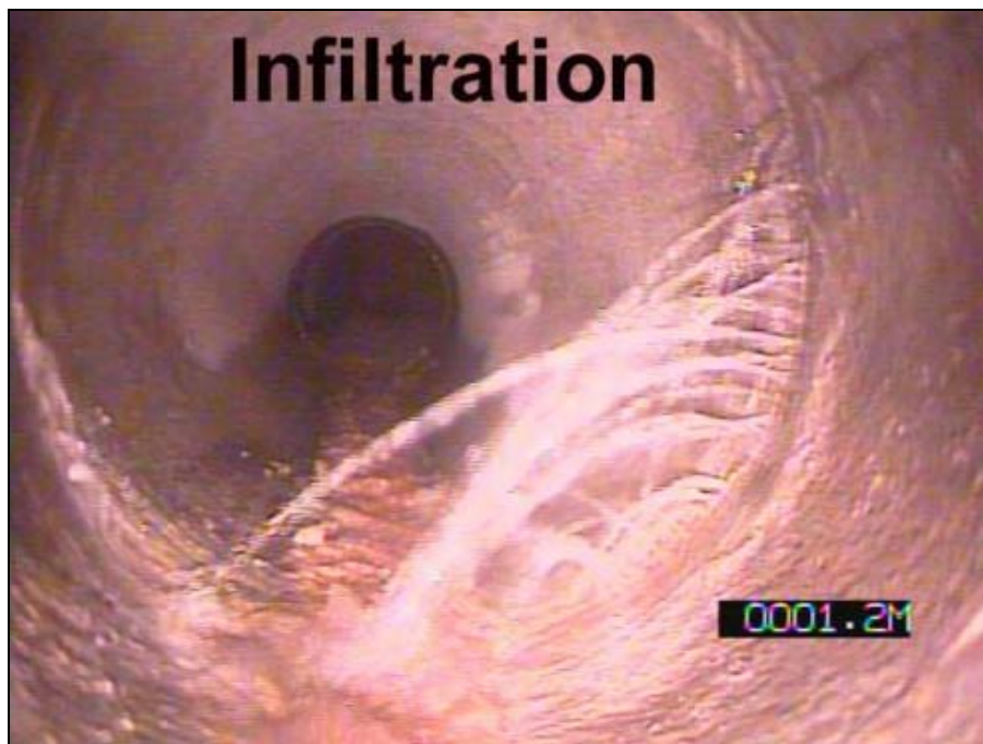
Figure 9.97 Example of infiltration into a sanitary sewer network (courtesy City of Surrey, Canada)
