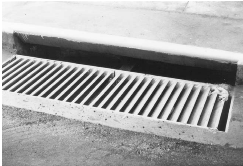
Figure 7.28 Combination curb opening & grate inlet (with 45 degree tilt-bar grate)
