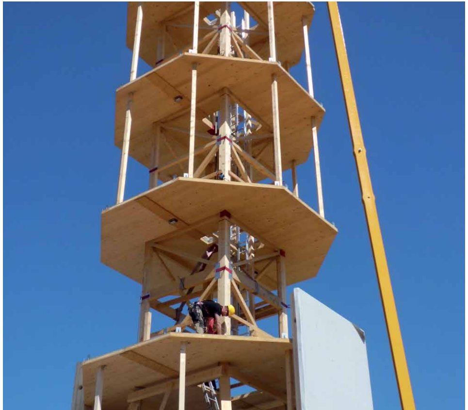
Tower scaffold - Image courtesy of TimberTower.
