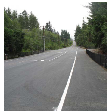
New left-turn lanes and shoulders on 180th Street SE improve traffic flow and safety
