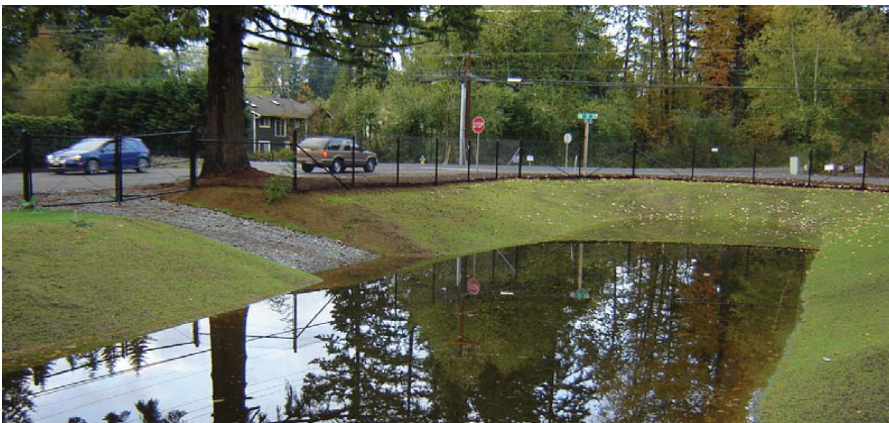
View from the southeast corner of the finished pond. Images courtesy of Snohomish County Department of Public Works.
