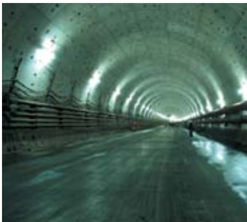
Chongming Tunnel. Image courtesy of AECOM.
