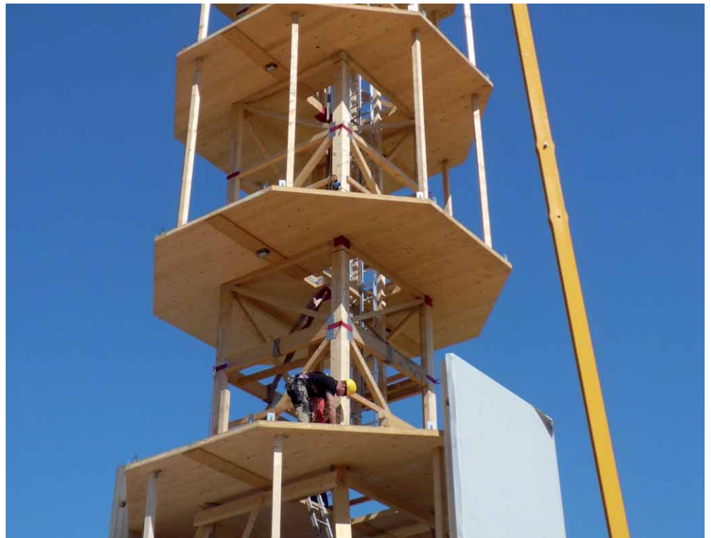
Pilot tower 1: Tower scaffold.
