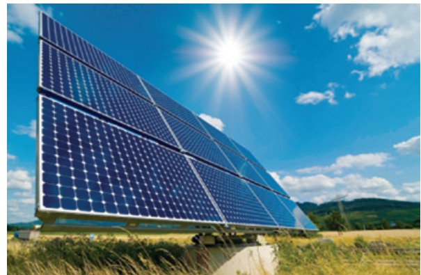
Gila Bend Solar Plant
