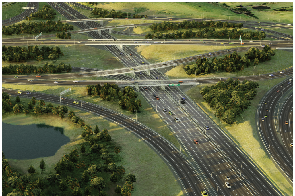
Aerial view of a highway with wireframe overlay. Designed in AutoCAD® Civil 3D® software. Rendered in Autodesk® 3ds Max® software.
