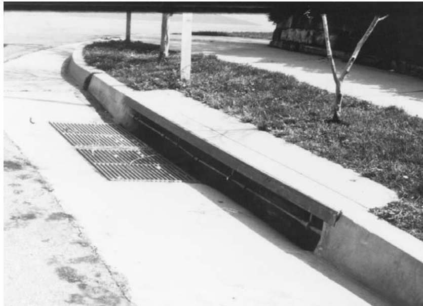
Figure 7.29 Combination sweeper curb opening & grate inlet
