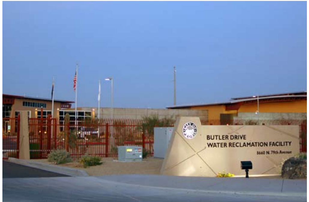
Butler Water Reclamation Facility: Entrance.
