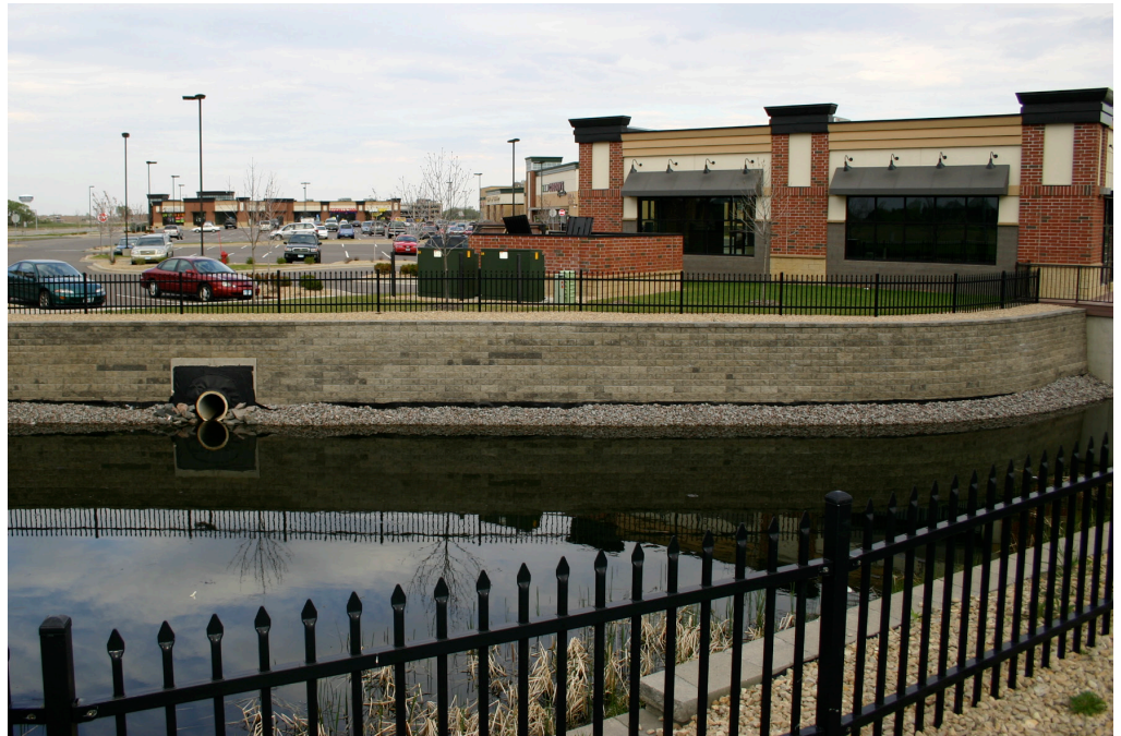
Typical commercial detention basin and development in Ramsey. Image courtesy of Bolton & Menk, Inc.
