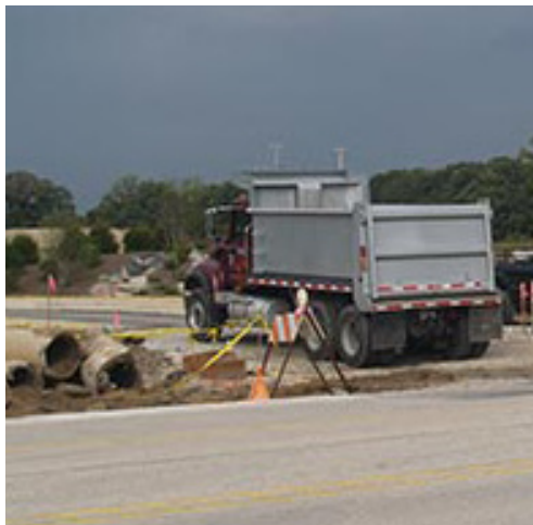
Storm sewer construction at Brookwood Farm. Image courtesy of Greengard, Inc.
