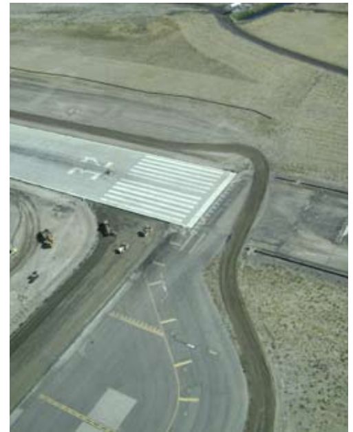
Taxiway G reconstruction.
