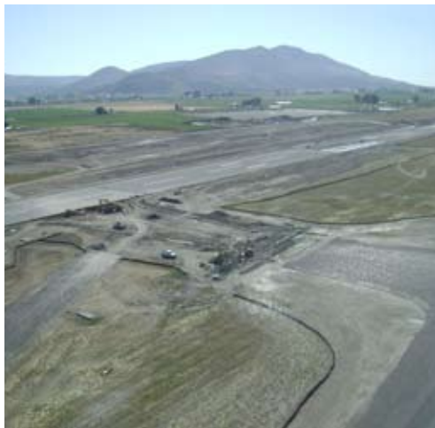
New Taxiway K under construction.
