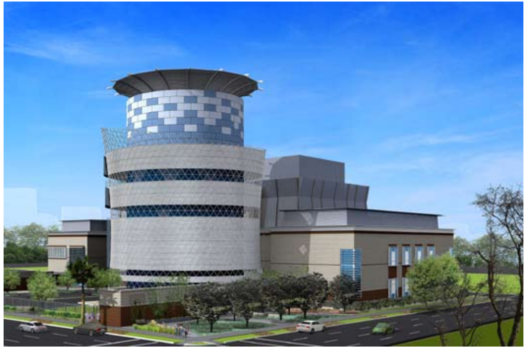
Sacramento Central Plant: Exterior
