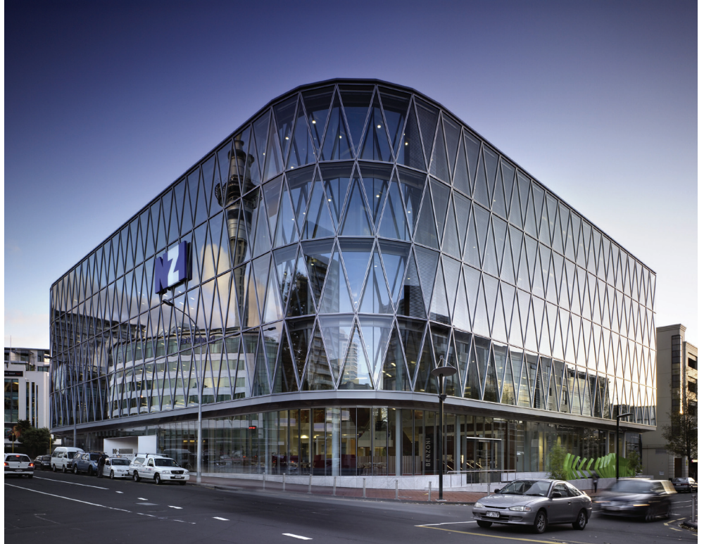
NZI Building, Fanshawe Street, Auckland.
