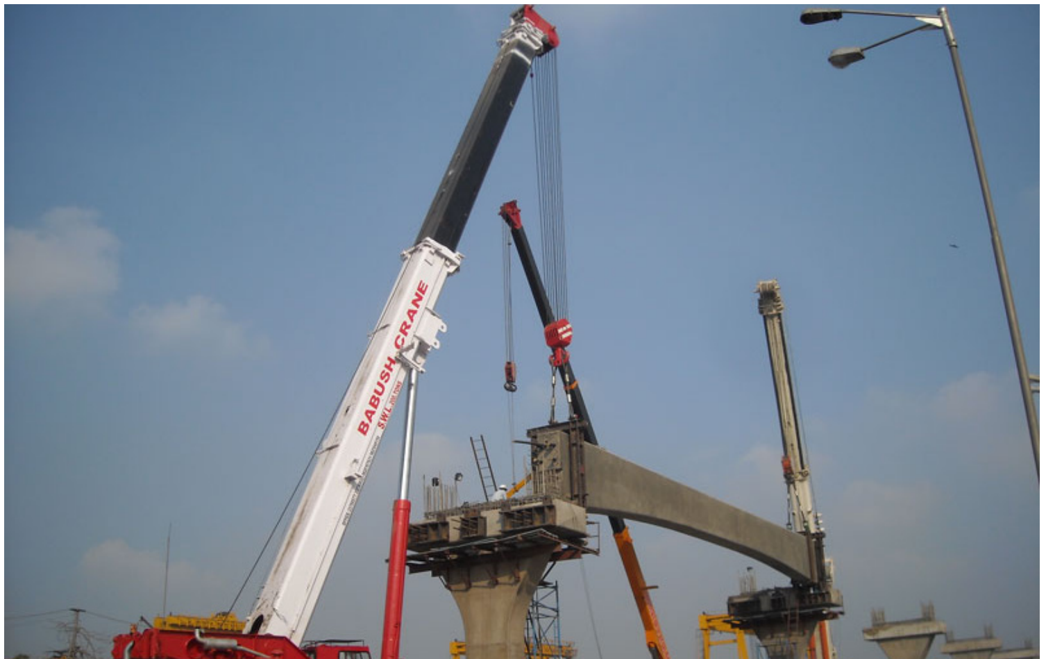
The first beam being lifted into place. Image courtesy of Larsen & Toubro.
