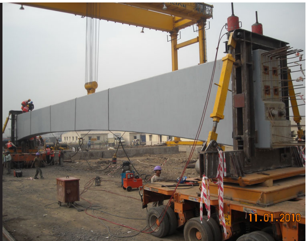
One of the first monorail beams for a new system: a beautiful sight for monorailists. The flat sided beam is being attached to special trailers for transportation to the monorail alignment. Image courtesy of Larsen & Toubro.
