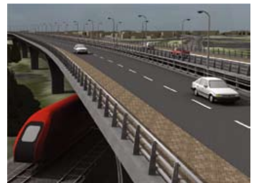
Image courtesy of Tibi Architects and RDV Systems
