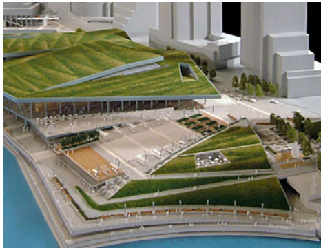
Vancouver Convention Center Expansion Project
