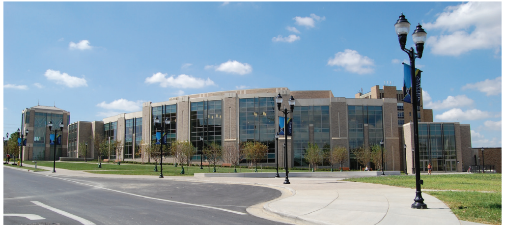
Conaton Learning Commons at Xavier University was designed and constructed using BIM processes.
