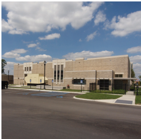
Messer developed building models of the 20,000-square-foot Central Utility Plant to aid construction.
